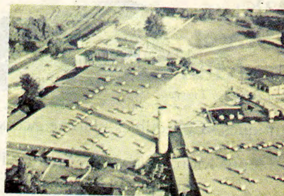
This is an aerial view of the mill that used to occupy the space that is now Town Hall and Food Lion.
