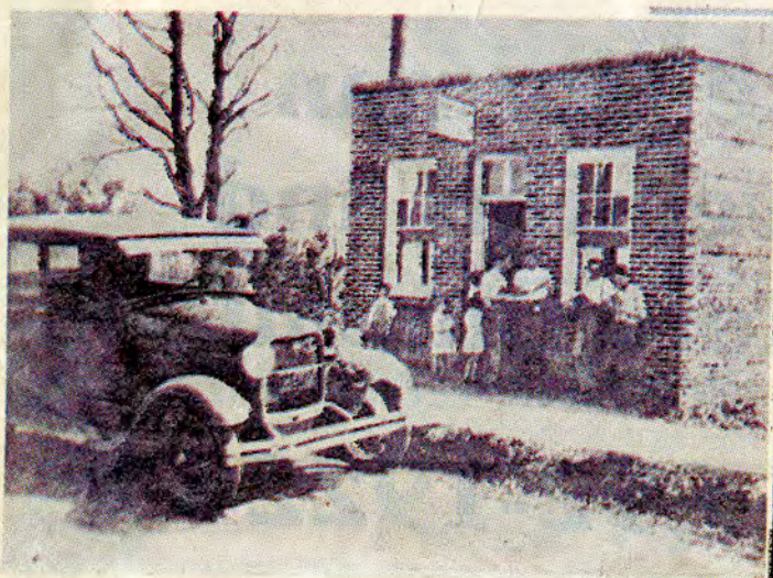
This is a photo of the Cornelius Town Hall and Library from around 1934.
