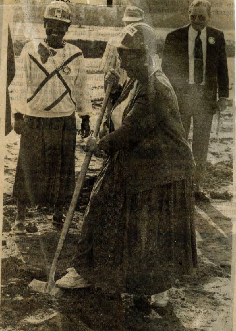
THE FIRST SHOVELFUL-- Vicki Hamilton, principal of Davidson Elementary School, breaks ground at the site of the new school. (Photo by Ed Decker)
